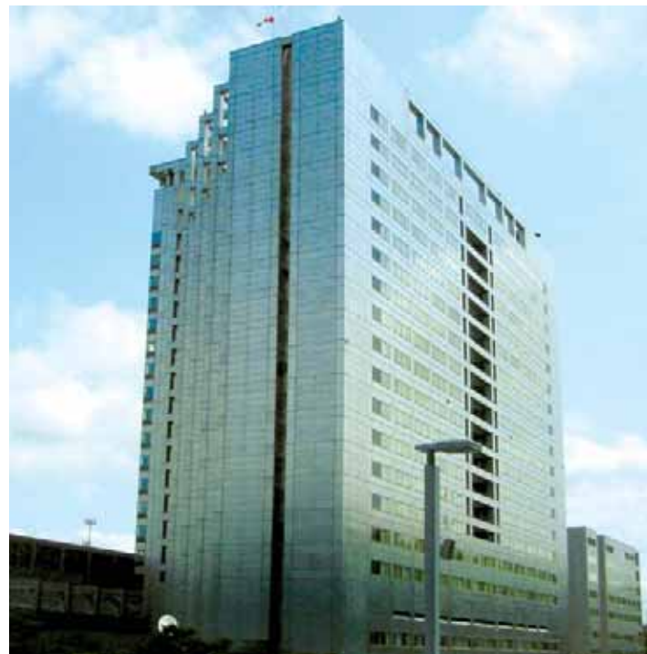
Samsung Medical Center, Seoul, South Korea Architect: Samoo Architects and Engineers, 1995 Aluminum stiffeners bonded to aluminum panels.
