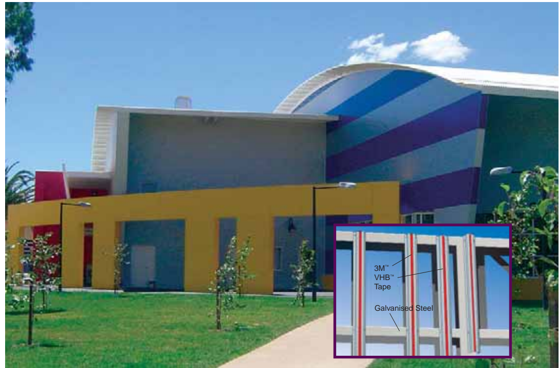
Canberra International Sports Centre Canberra, Australia Architects: Peter Hunt Architects, 2004 Builder: Sports Centre Australia (Konstantinou Group) Composite panels to gal top-hats.
