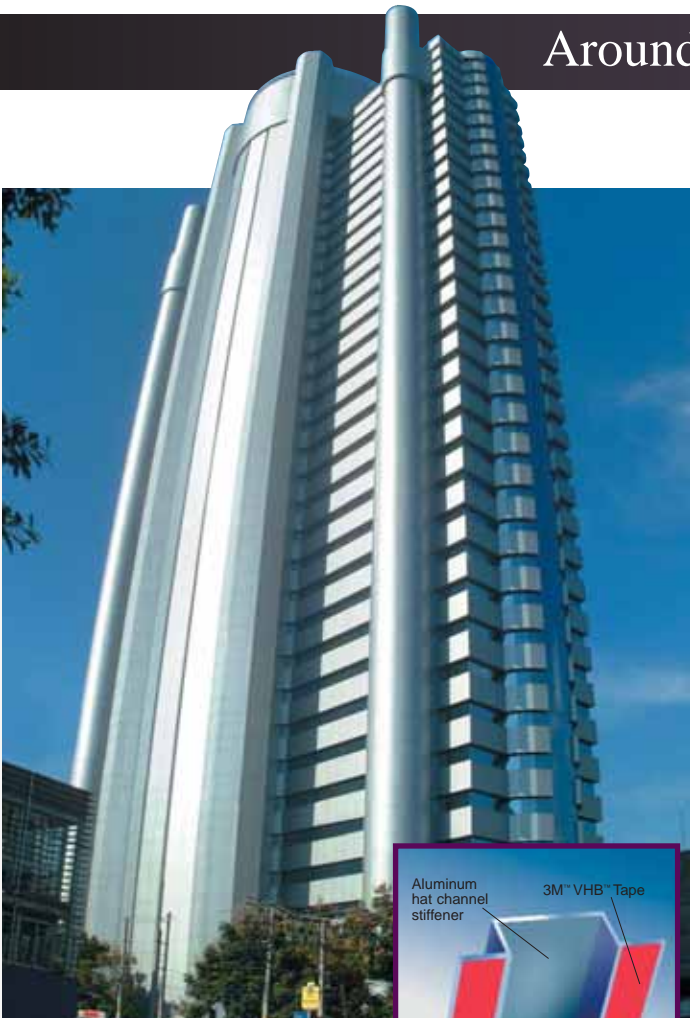
Plaza Centenário, Sao Paulo, Brazil Architect: Carlos Bratke, 1995 Aluminum stiffeners bonded to ACM panels.
